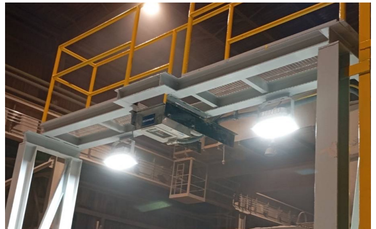
AMI'S IOCONVEYOR® INSTALLATION
